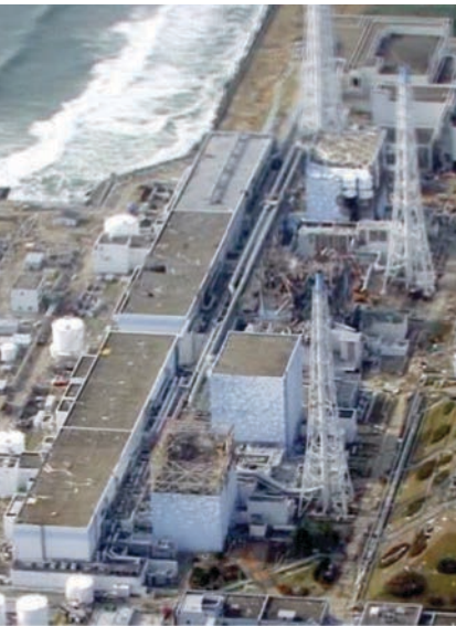
▲ In 2011, the Fukushima Daiichi Nuclear Power Plant in Japan overheated as a result of a 9.0 magnitude earthquake that triggered a tsunami that flooded the coastal plant and caused the cooling system pumps to fail.
